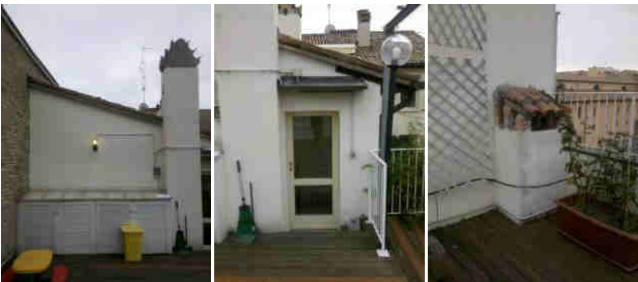
Figure 9: from left to right: the cabinet, the access and the small chimney
