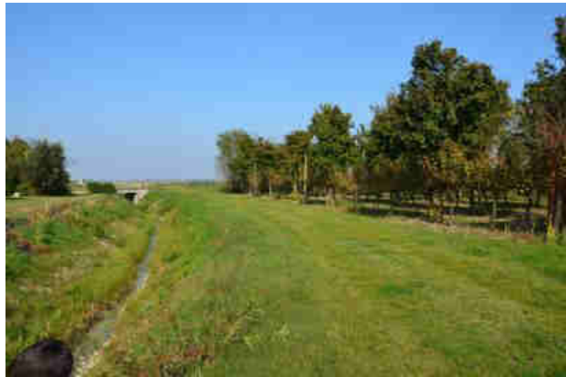
View of the Irrigation canal on the West side
