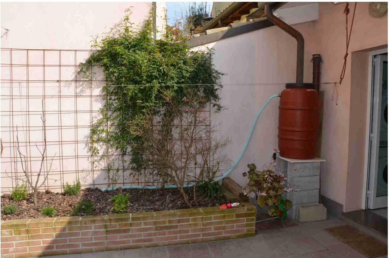
Figure 6: Rain water collected from the roof and stored in a tank. From the tank to the dripping line system.
